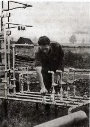
"A twist of the wrist and I regulate pressure in oil sands far below the earth's surface," says Floyd Williams as he turns a controlling air-valve, on a Pennsylvania well. Modern re-pressuring operations in oil producing areas in Pennsylvania have renewed many old wells, and made new ones flow faster—to the everlasting advantage of your car and your pocketbook.
